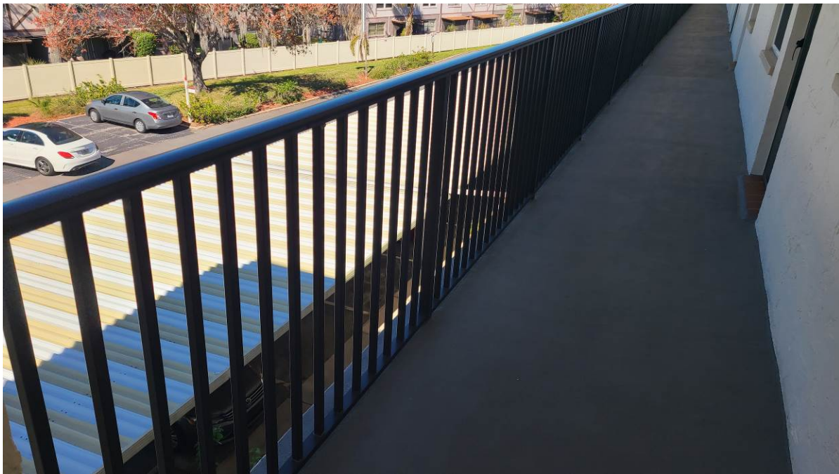
Photograph 7: Building Walkway and Guard System (3 rd Level)
