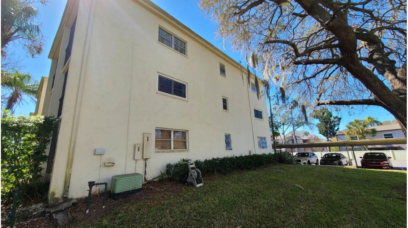
Photograph 3: View of the North Elevation of the Condominium.
