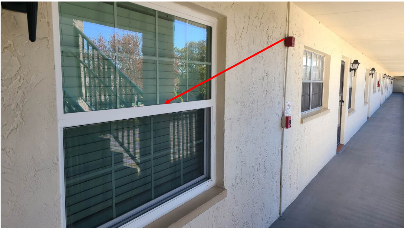
Photograph 10: Unit Windows – Appear Replaced
