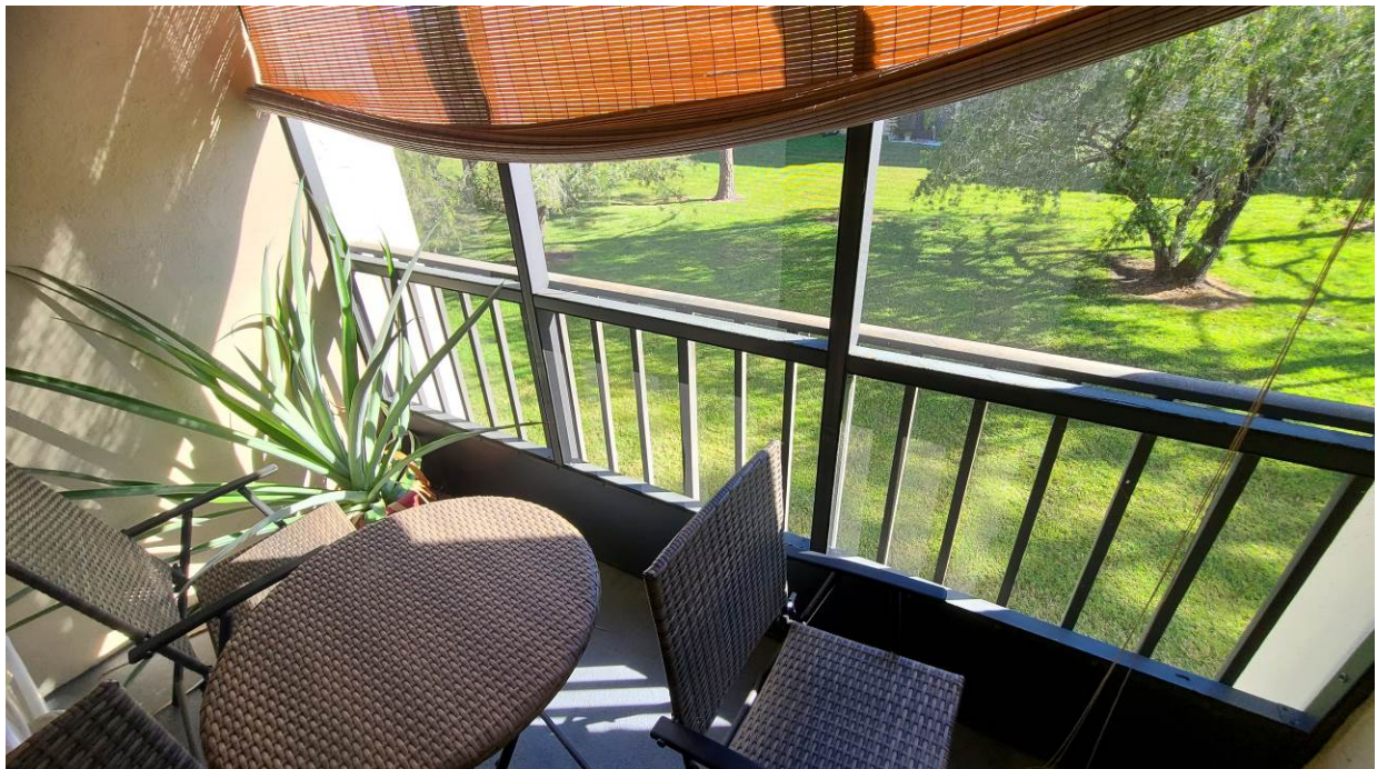
Photograph 6: Unit #206 Balcony, Guards and Enclosure System
