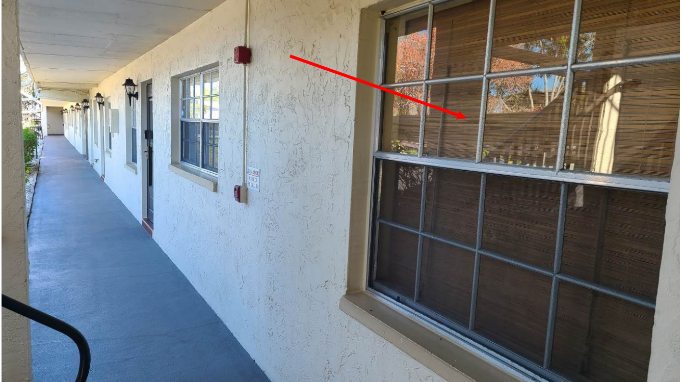
Photograph 9: Unit Windows – Appear Original
