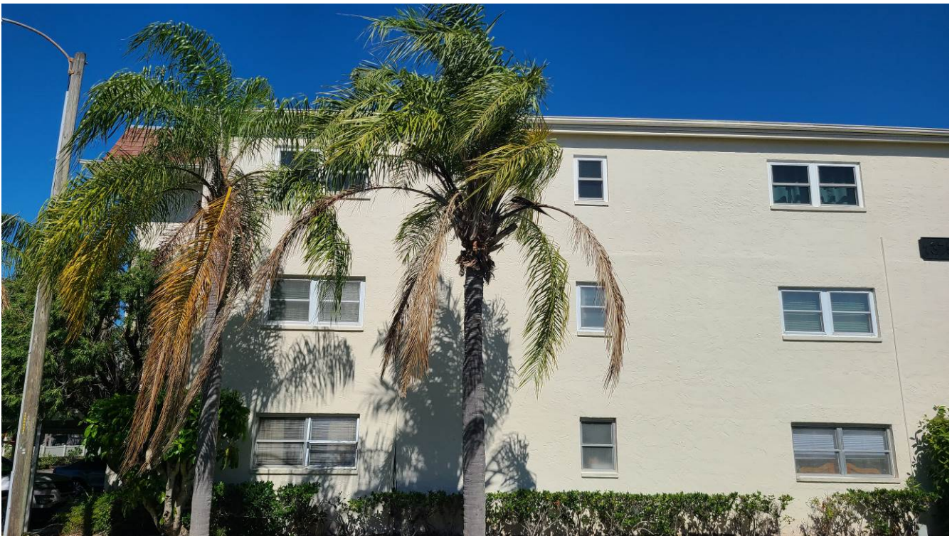
Photograph 4: View of the South Elevation of the condominium.
