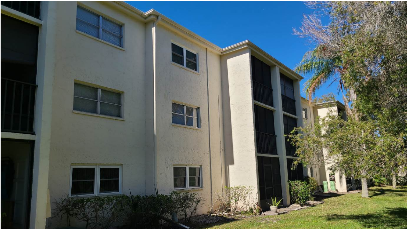
Photograph 2: View of the East (Back) Elevation of the Condominium.
