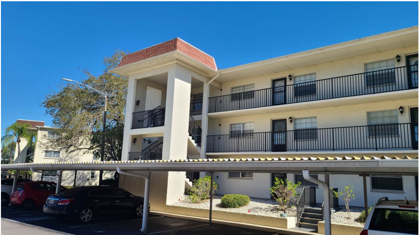
Photograph 1: View of the West (Front) Elevation of the Condominium.
