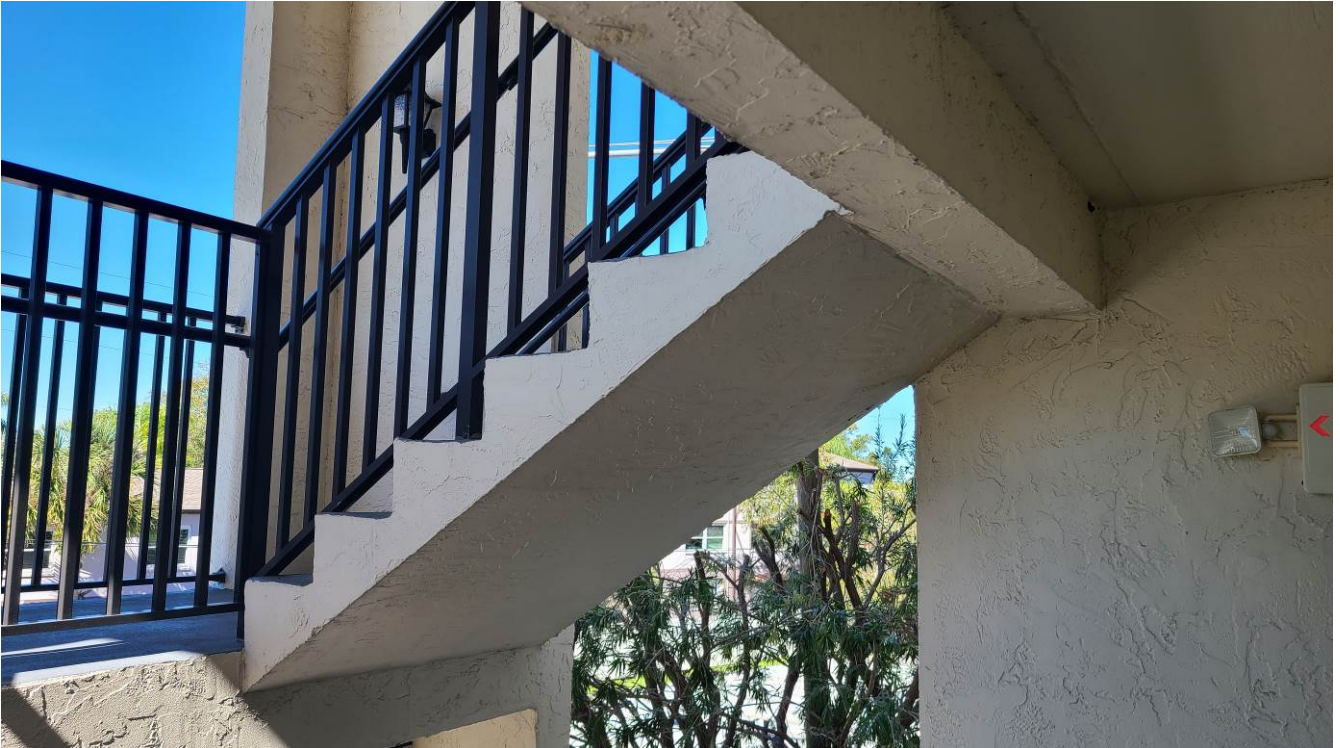
Photograph 8: Building Staircase (North End)
